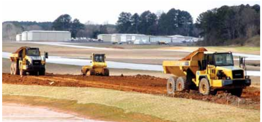
A crew at Pittman Construction's Covington, Ga., airport project hauls dirt with two Komatsu HM300-2 haul trucks and grades the site using a Komatsu D65-17 dozer. The company owns more than 30 Komatsu machines.
